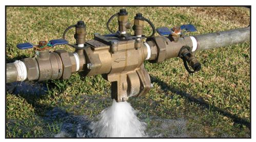
The opening point of the relief valve is determined, in part, by the relief valve spring. The springs are designed to operate within specific tolerances. They may vary slightly from one spring to the next. After some initial use, the spring will "set" or settle in at a fairly consistent point. However, one may still find that the relief valve opening point changes.
